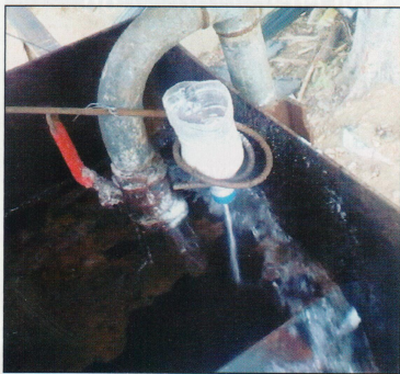
Mixing polymer for stabilisation
